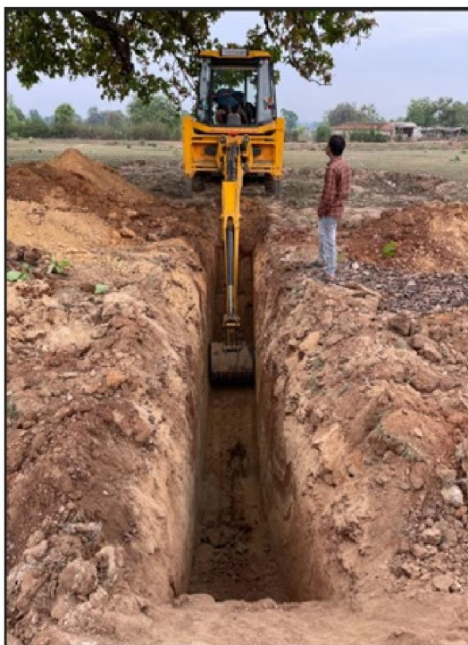
Field Photo-10.1: Photograph showing Excavation of Trenches (T3, T5) and Trench mapping sampling work, Sitapur Block
