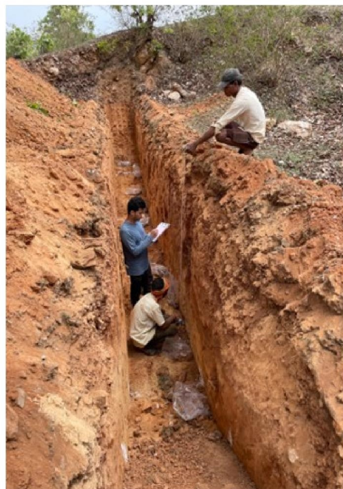
Field Photo-10.1: Photograph showing Excavation of Trenches (T3, T5) and Trench mapping sampling work, Sitapur Block
